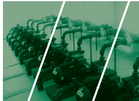
Boosting and Distribution of surface water
